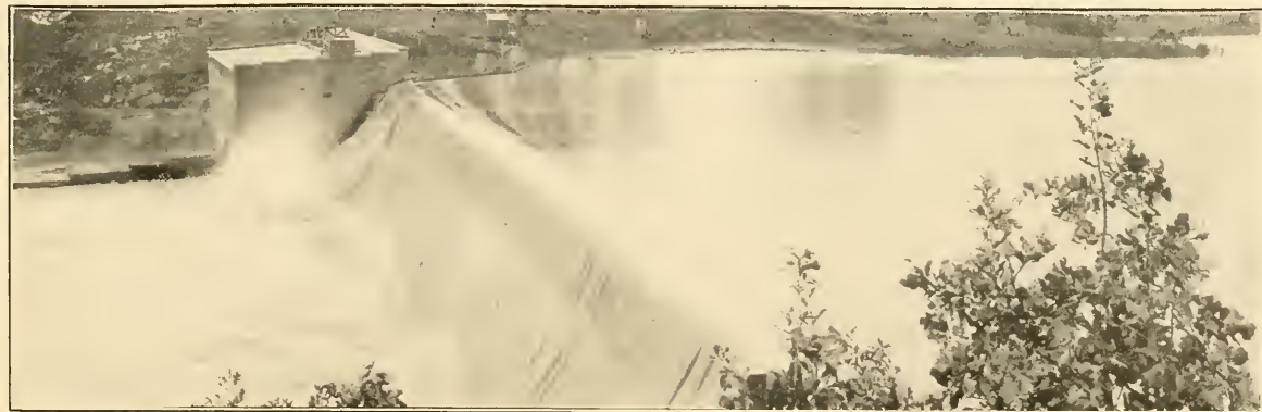
RIVER SCENES. (1) Tallapoosa which joins the Coosa above Montgomery, forming (2) the Alabama which flows 320 miles into the Mobile. TALLASSEE FALLS, 30 miles above Montgomery, and power house of the Montgomery Light & Water Power Company, where 8,000 horse power is developed for lighting and manufacturing purposes in the city, giving Montgomery the lowest rates in the South for light and power.
